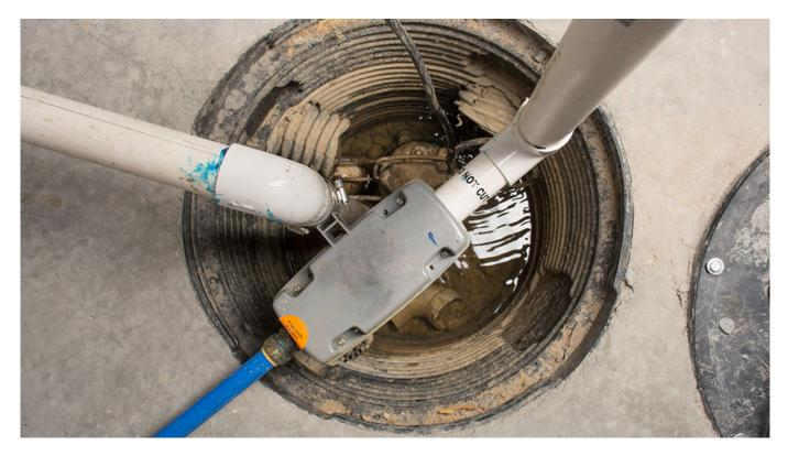
A sump pump prevents water damage by taking excess water from your basement and pumping it out of your house. However, without regular maintenance, it may malfunction – causing water to overflow and damage your home. To keep your sump pump running smoothly, proper upkeep is essential. Help extend its life, prevent costly repairs or replacements, and even reduce your energy bills by following along with our sump pump maintenance checklist.
