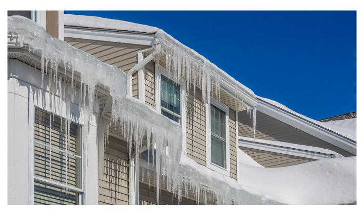
When winter weather arrives, you're used to shoveling, snow blowing, salting the sidewalks, and scraping windshields. But beyond those building and vehicle precautions, there is an additional winter threat to watch for. Ice dams can appear on a roof over time as snow and ice melt and refreeze during the winter months. The resulting ice masses on your gutters or roof's edge aren't just a threat to your home or business, they can also be dangerous for anyone standing below them.
